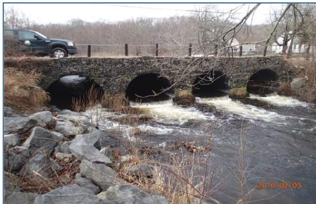
View of Walnut Street crossing in Essex over the Falls River. The four perched corrugated metal culverts (left photo) were replaced with a clear span bridge (right photo).
